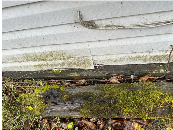
Moisture Intrusion - Downspout
